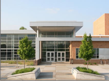
MAIN ENTRANCE ON THE NORTH SIDE OF THE BUILDING
